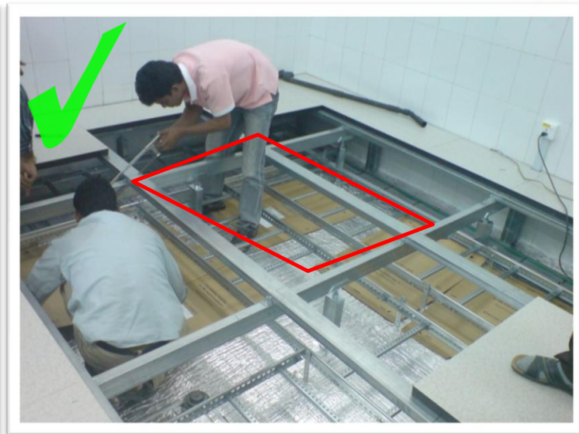
Use paper over insulation during installation
